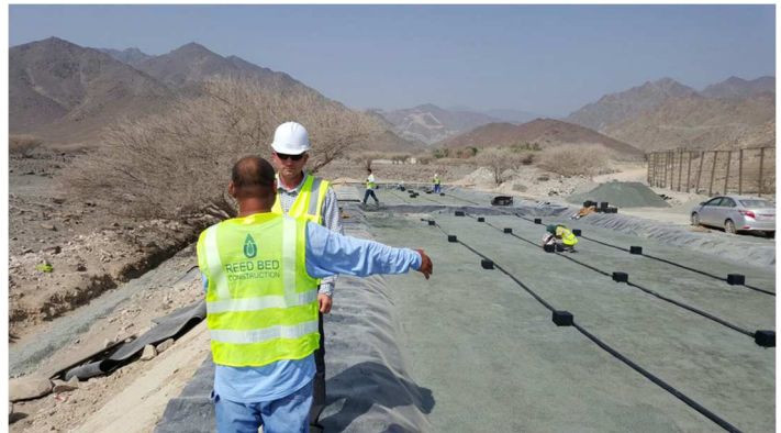
Installation of distribution pipes
