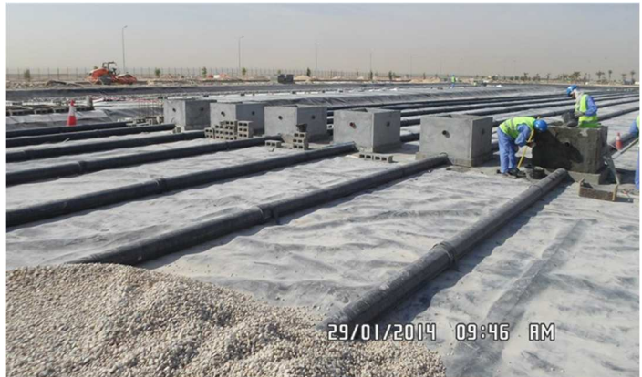
Drainage system and gravel filter
