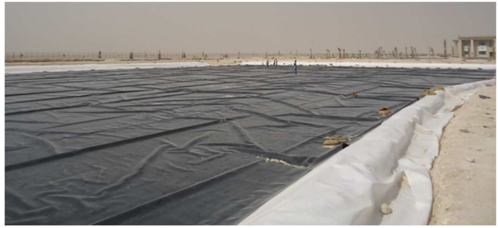
Liner installation
