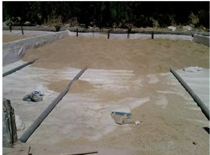
Filter layer installation
