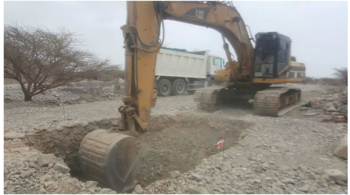
Excavation septic tank
