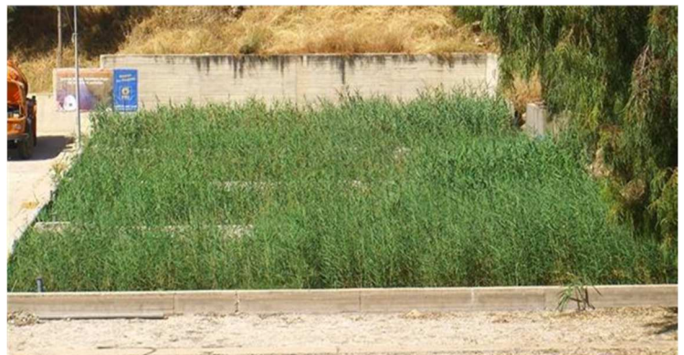
Sludge bed 7 months under operation (Oct.- Mai)
