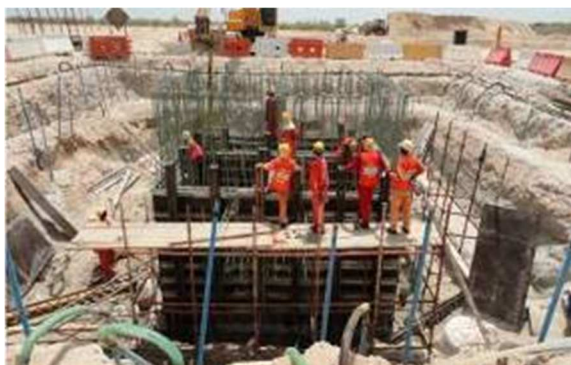
Casting pump station
