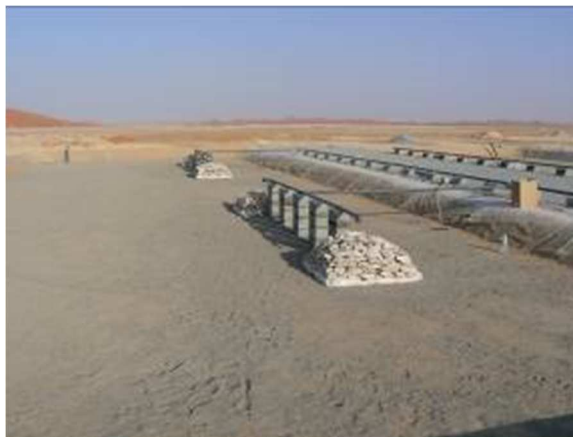
Reed bed 1. stage, under construction
