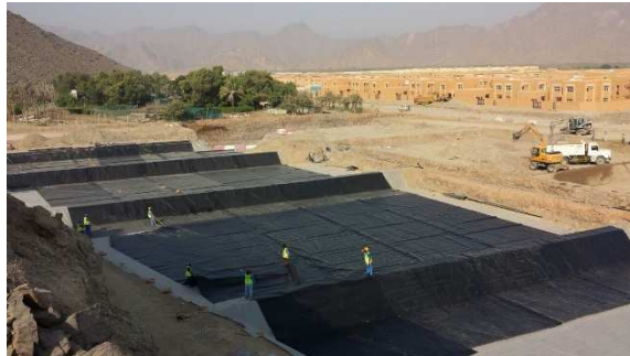
Liner installation
