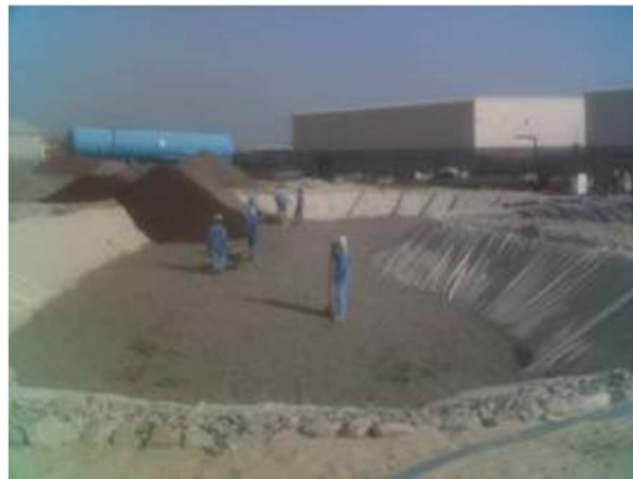
Filling of filter material
