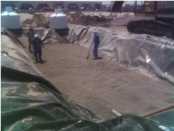
Filling of filter material
