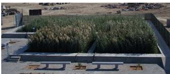
Reed Bed treatment system after 6 months of operation
