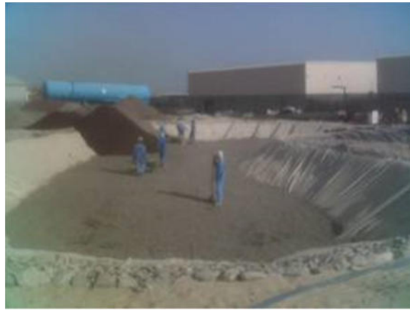
Filling of filter material
