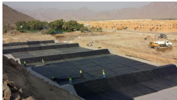
Liner installation
