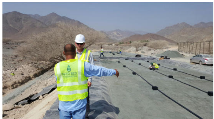
Installation of distribution pipes
