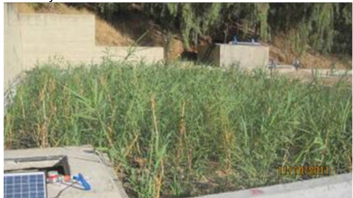
Sludge bed 2 months under operation
