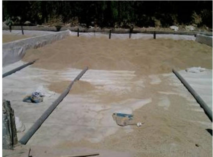
Filter layer installation
