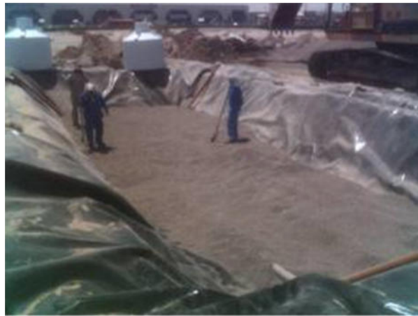
Filling of filter material
