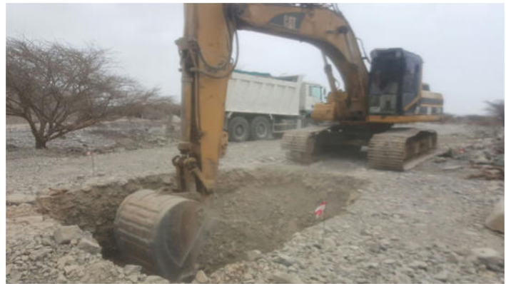
Excavation septic tank
