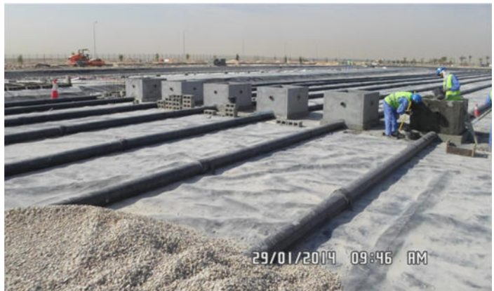
Drainage system and gravel filter
