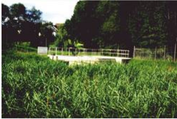
Picture of a retention planted soil filter
