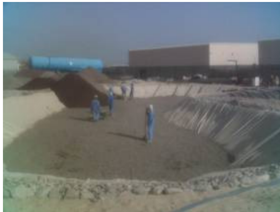
Filling of filter material
