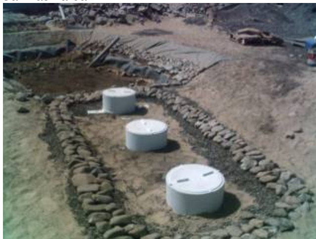
Oil separator and fresh planted reed bed
