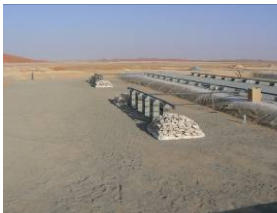
Reed bed 1. stage, under construction
