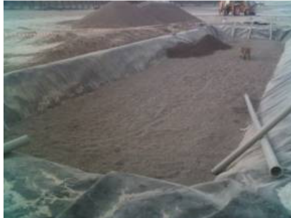
Filling of filter material
