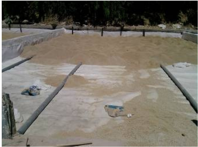
Filter layer installation
