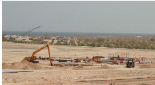
Excavation of pump station
