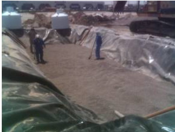
Filling of filter material
