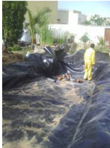
Installation of liner
