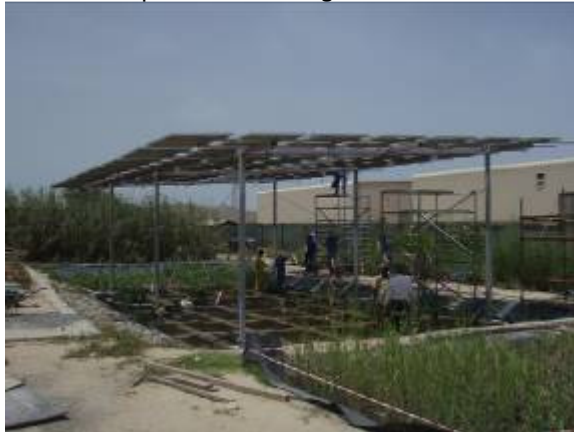
Vertical flow reed bed after reed harvesting and installation of solar panels above reed bed
