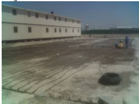
Installation of subsurface drip lines
