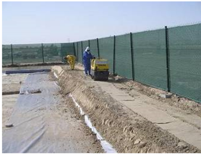
Installation of dams
