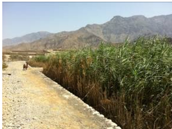
Basins after 1 year of operation
