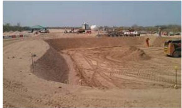
Excavation of basins
