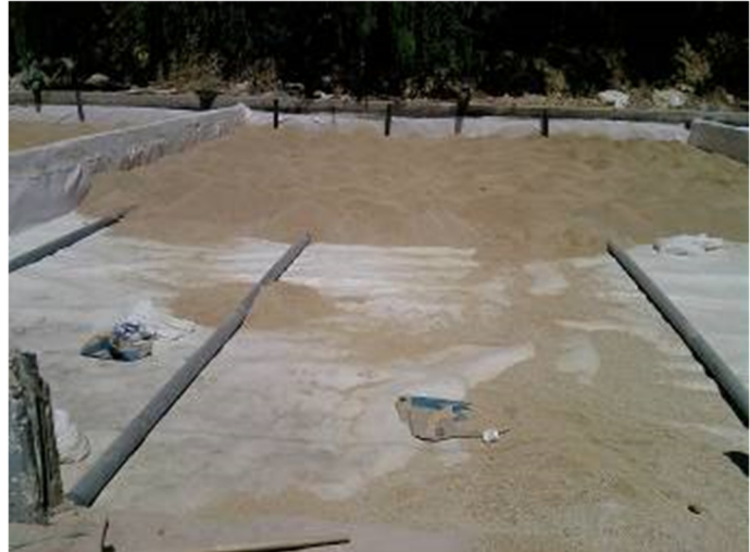
Filter layer installation
