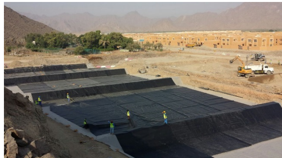
Liner installation
