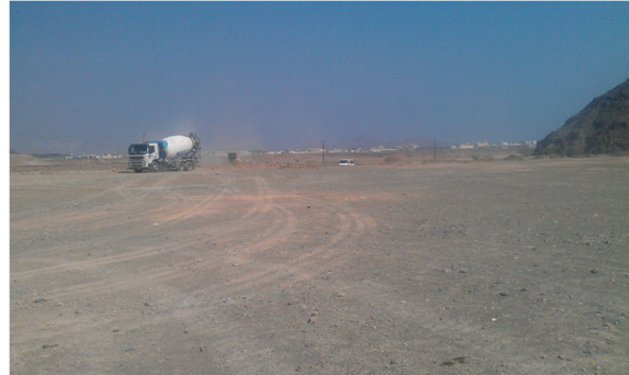
Start of excavation and filling
