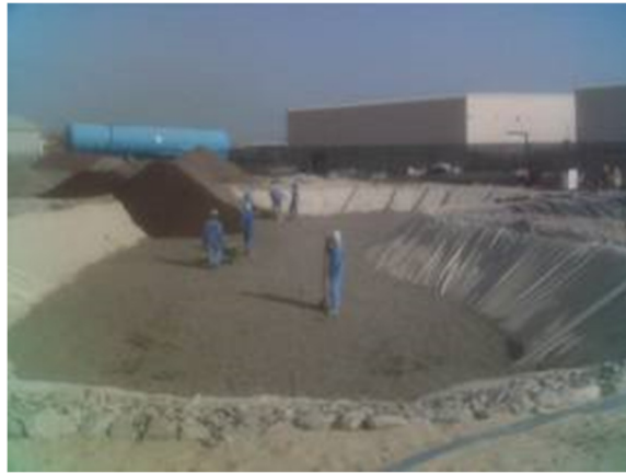
Filling of filter material
