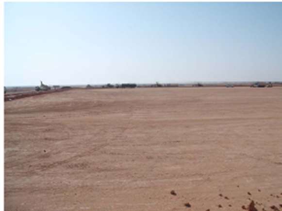
Basins under construction
