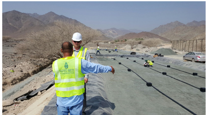
Installation of distribution pipes
