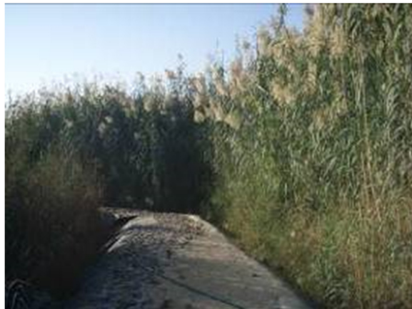
Reed Bed after 1 year of operation
