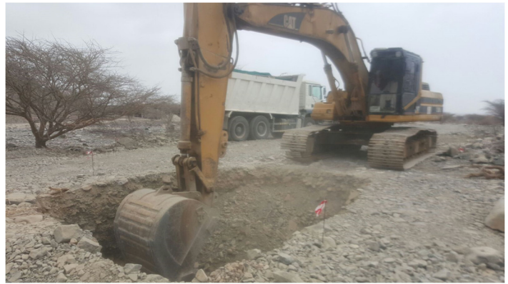
Excavation septic tank
