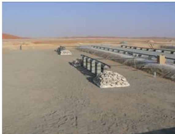
Reed bed 1. stage, under construction
