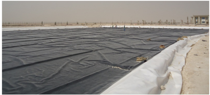
Liner installation
