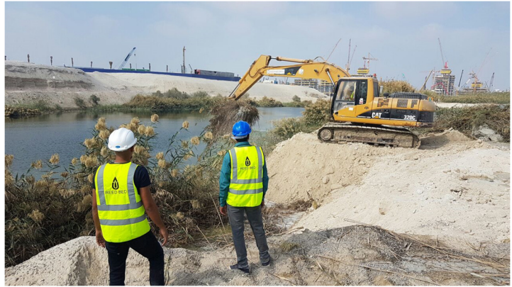
Excavation of reed plants
