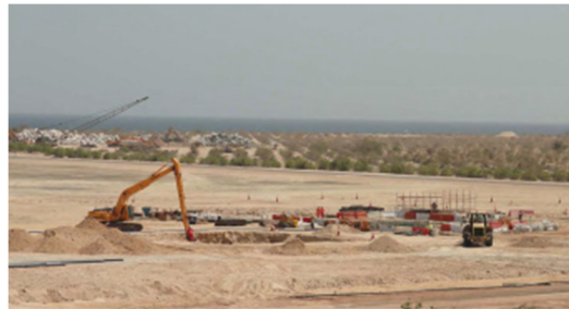
Excavation of pump station
