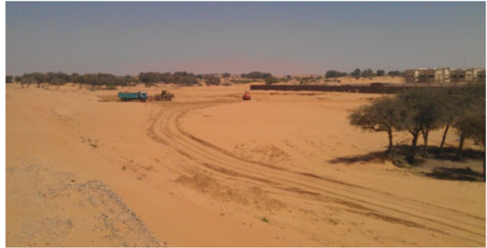
Start of excavation and filling
