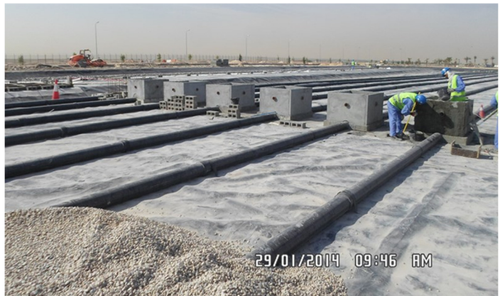
Drainage system and gravel filter
