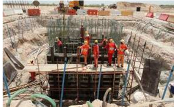
Casting pump station
