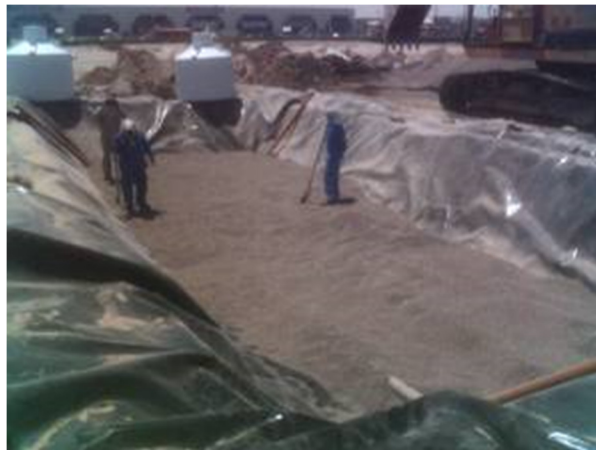
Filling of filter material
