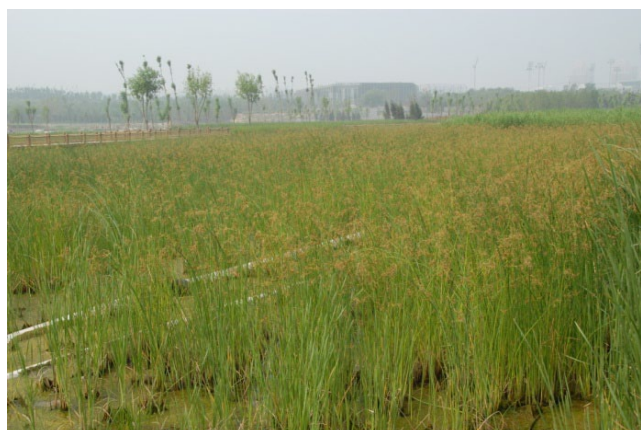
Figure 12. Simsen ( Scirpus sp. ) in a VFB treating domestic wastewater in the Olympic Forest Park in Beijing, China (photo by J. Germer, 2008).
