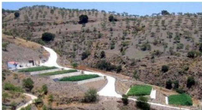
Figure 24. French System, from left to right: three VFBs (filters) for pre-treatment and two VFBs for secondary treatment in Albondón, Spain, with 800 inhabitants. The plant needs no electricity supply as it is built on a slope (photo by T. Burkard, 2005).
