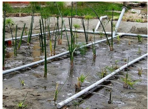
Figure 6. VFB under construction, during influent pumping with greywater to test for uniform distribution in Lima, Peru. Note the small holes in distribution pipes. The entire surface is used as an inlet area, and the pipes are later covered with gravel after completing the testing (photo by H. Hoffmann, 2008).
