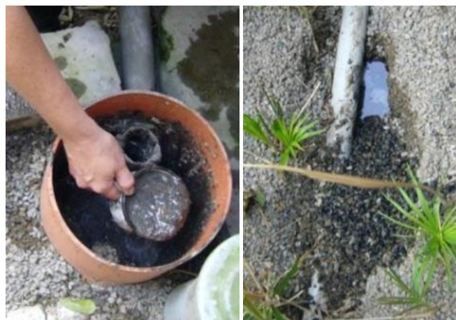
Figure 28. Left: Malfunctioning grease trap with too much sludge accumulation. Right: the sludge from the grease trap obstructs the infiltration area of the CW which has become black because there is no oxygen transport anymore and it has become clogged (photo by H. Hoffmann, 2009).
