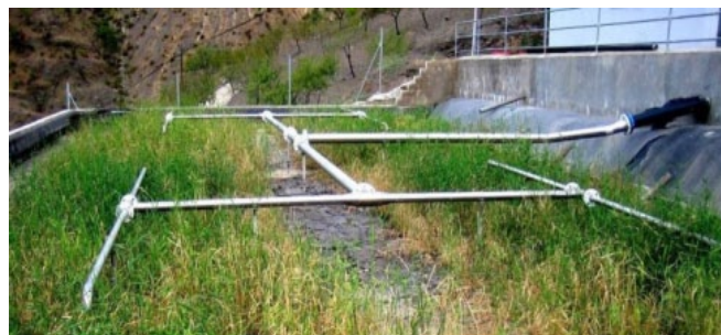
Figure 26. Distribution pipes for raw wastewater in first stage (VFB) in French System in Albondón, Spain (photo by T. Burkard, 2007).
