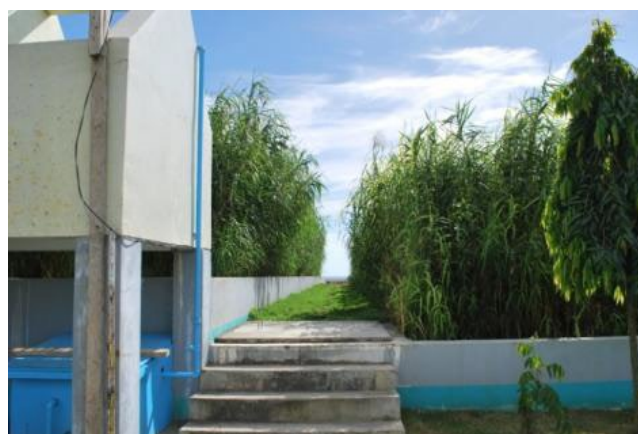
Figure 27. Subsurface flow CW in Bayawan city, Philippines. The path in the middle separates the VFB and the HFB (photo by J. Boorsma, 2009; project supported by GIZ) 24 .
