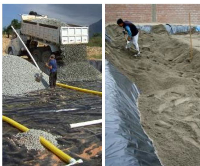
Figure 9. Left: VFB during construction in Palhoça, Santa Catarina, Brazil; drain pipes situated on top of the PE liner are being covered with gravel. Right: VFB in Lima, Peru during filling with sand (photos by H. Hoffmann, 2007).
