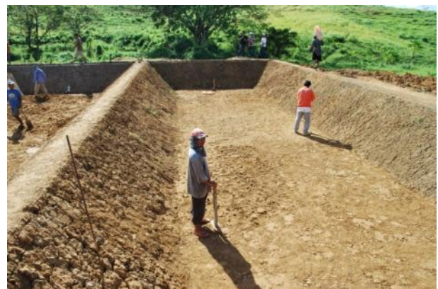
Figure 7. VFB under construction in Bayawan City, Philippines; the wetland will treat wastewater from a landfill (photo by J. Boorsma, 2009; project supported by GIZ).
