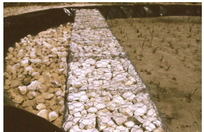
Figure 20. Inflow zone with stones in a HFB near Leiria, Portugal (photo by J. Vymazal, 2003).
