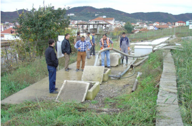
Figure 13: Pumping of settled sludge from pre-treatment unit of subsurface flow CW in Tirana, Albania. The removed sludge will be taken to a local wastewater treatment plant by tanker (project supported by GIZ, photo by J. Nowak, 2010)
