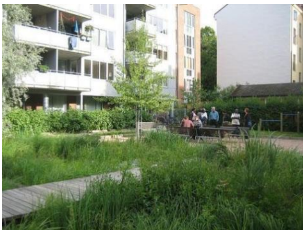
Figure 2. Urban decentralised greywater treatment with a subsurface flow CW in Klosterenga in Oslo, Norway (photo by L. Ulrich, 2008).
