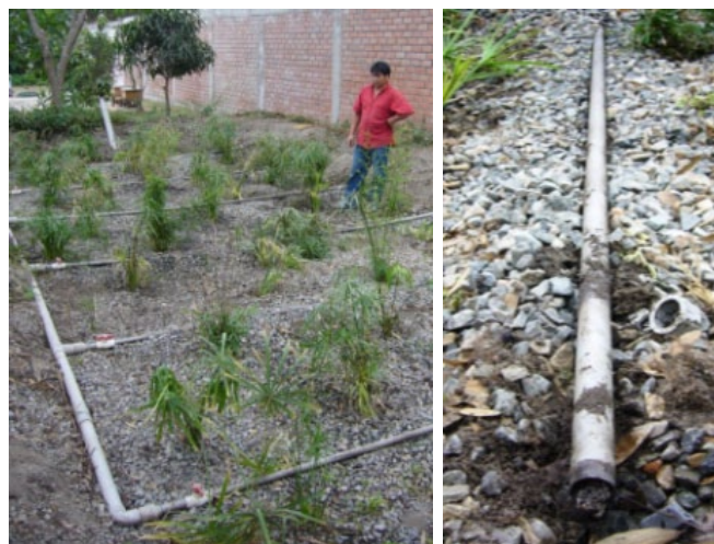
Figure 29. Left: cleaning the wastewater distribution pipes by opening and closing valves and caps during the pumping phase (medium sized papyrus umbrella sedge plants just after re-planting). Right: opened cap on a blocked distribution pipe (photos of VFB for blackwater treatment at school in Lima, Peru by H. Hoffmann, 2009)
