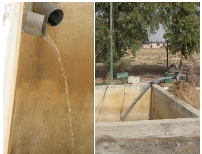
Figure 3. The treated effluent (left) of the vertical flow constructed wetland in Haran Al-Awamied, Syria, is collected in this storage tank (right) before its reuse for irrigation in agriculture (photos by E. von Muench, 2009; project supported by GIZ).
