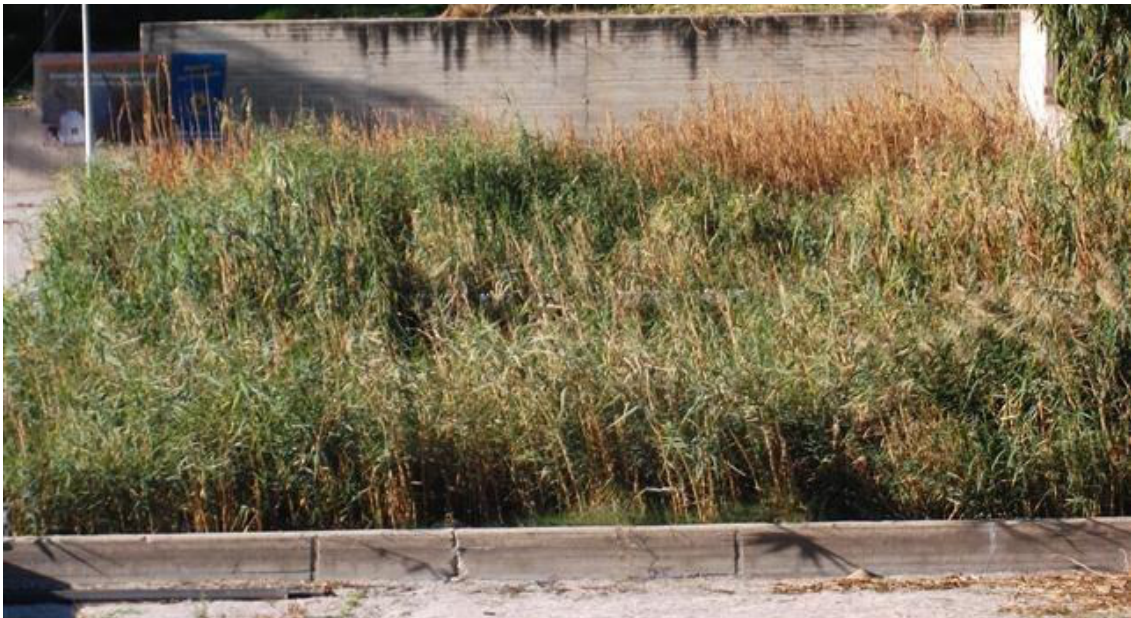
Sewage sludge dewatering in Al Salt, Jordan, Pilot System 4 x 160 m 2 , 2011-2013
