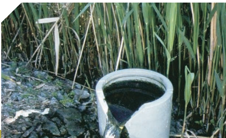
Submerged pipe inlet – riser pipes with V-notches (Cooper et al. , 1996)
