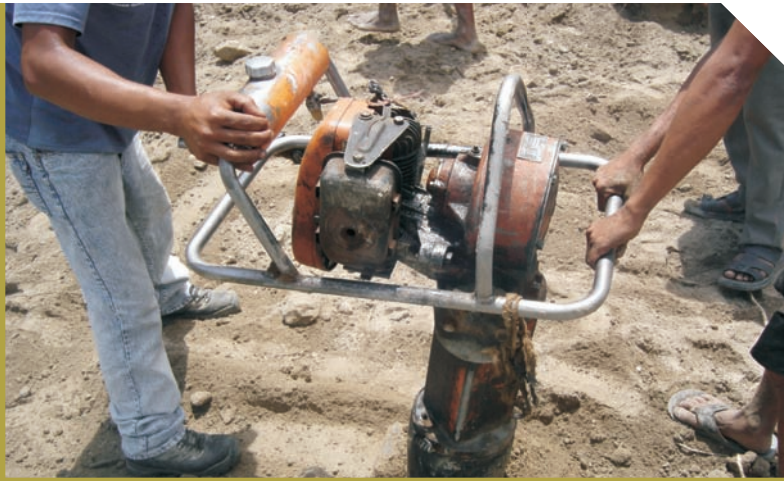
Compaction of the subgrade works
