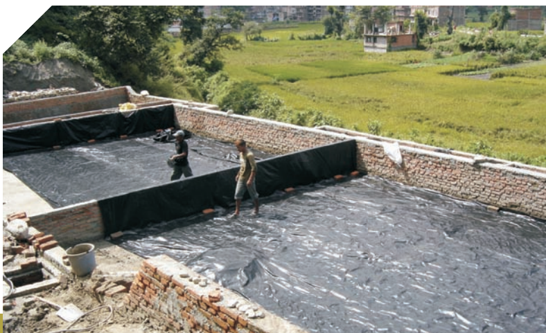
Plastic liners placed in the basin
