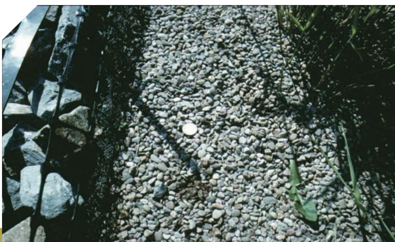
Gabion inlet (Cooper et al. , 1996)
