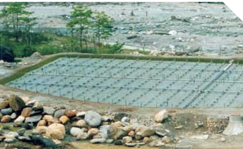
Vertical flow constructed wetland (Shrestha R.R.)
