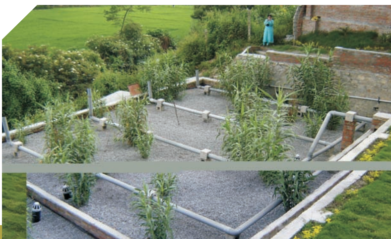
Pipe network inlet with main pipe in the edge
