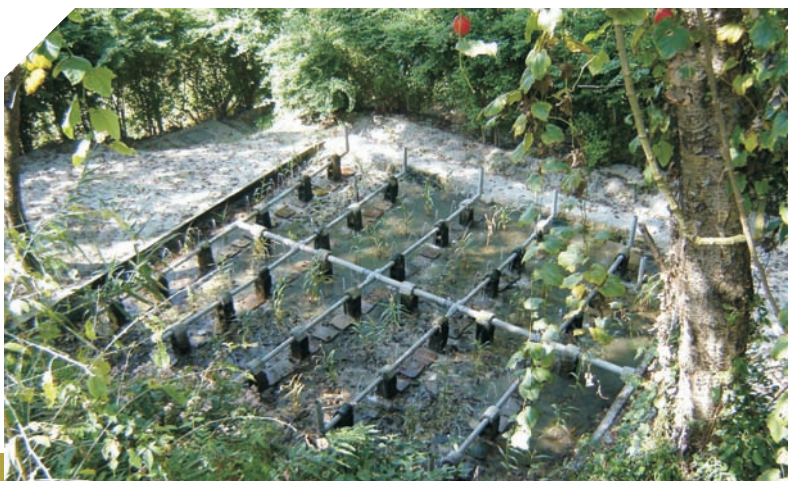
Pipe network inlet with main pipe in the centre
