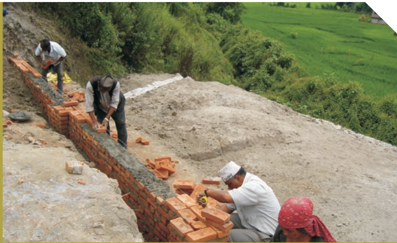
Construction of walls of the basin
