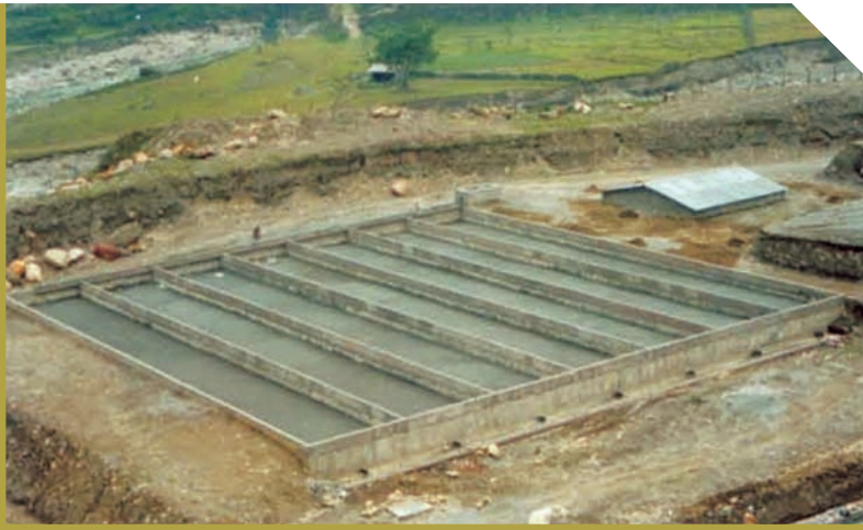
Sludge drying bed (Shrestha R.R.)
