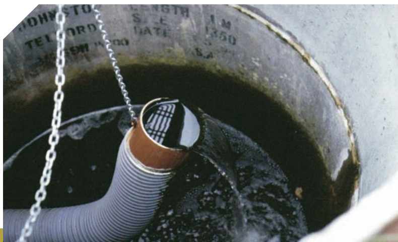
Flexible pipe outlet (Cooper et al. , 1996)
