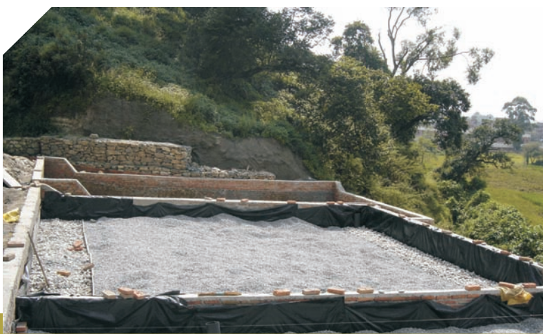
Filling substrate in horizontal flow CW (please note the inlet and outlet zones)
