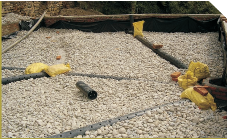
Installation of collection network and filling of substrate (drainage layer) in vertical flow CW
