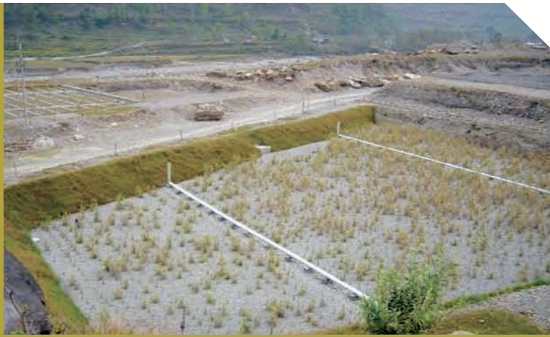
Horizontal flow constructed wetland (Shrestha R.R.)
