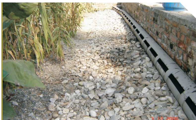
Slotted pipe inlet
