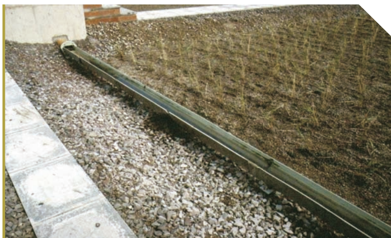
Channel inlet (Cooper et al. , 1996)
