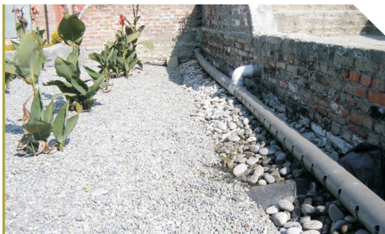
Perforated pipe inlet
