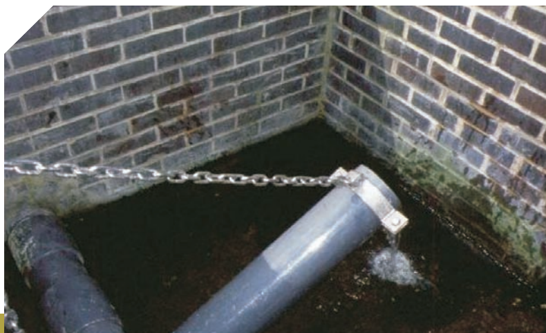
Swivelling elbow outlet (Cooper et al. , 1996)
